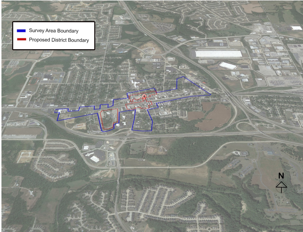
Figure1: Wentzville Intensive Survey. Context map including area of study and proposed historic districts, Source: Google Earth Pro. Web: Accessed 7 March 2022. Boundary and labels added by report authors. (38°48'40.2"N 90°51'10.5"W).
